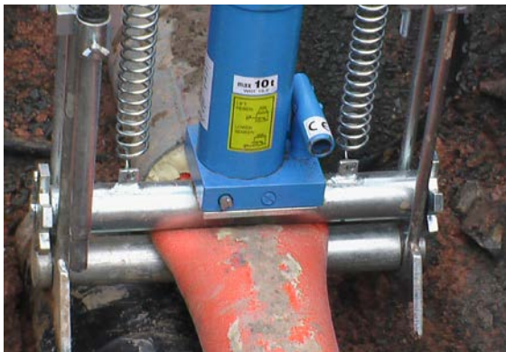
Fig. 07-31 Squeezing off UNO carrier pipes
