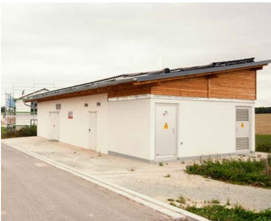
Heat source/energy centre
