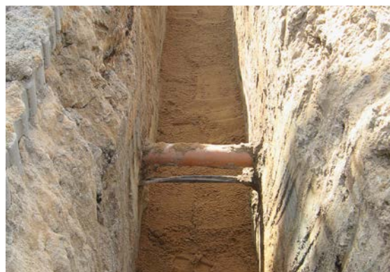
Fig. 07-2 Trench base with pipe support
