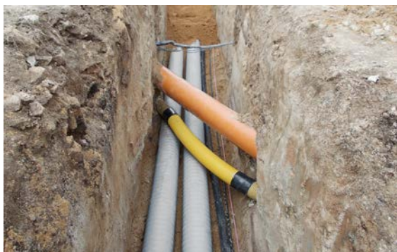
Fig. 07-22 Passing beneath crossing lines
