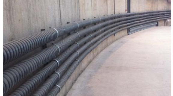
Fig. 07-28 Example of above ground / wall mounting
