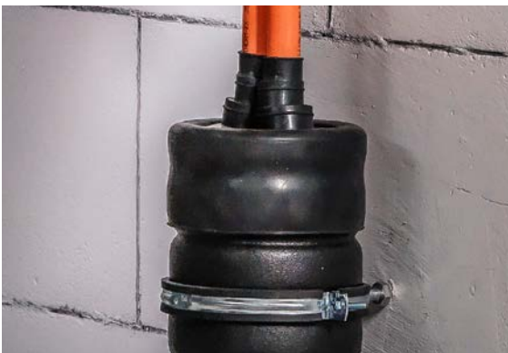
Fig. 05-23 Closing pipe with rubber end cap
