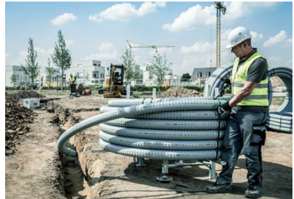
Fig. 07-34 Stationary horizontal pipe decoiler at the end of the trench
