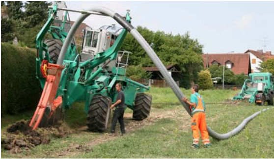
Fig. 07-8 Installation with mole ploughing machine
