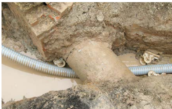
Fig. 07-24 Easy installation thanks to flexible pipe routing
