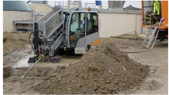
Fig. 07-10 Installation with horizontal directional drilling device
