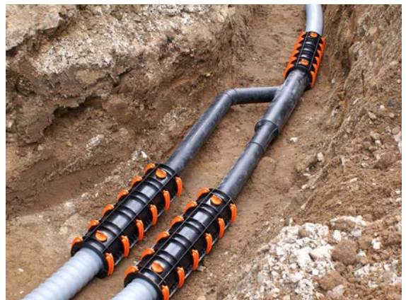
Fig. 04-34 Y-pipe installation in practice
