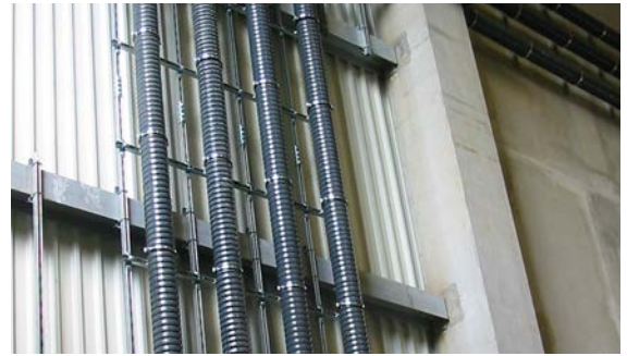
Fig. 07-29 Example of above ground/ wall mounting
