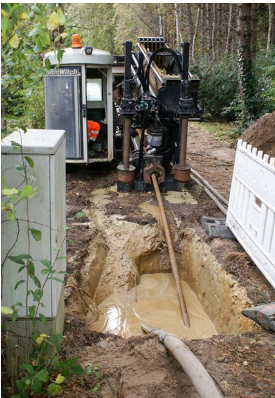
Fig. 07-13 RAUTHERMEX directional drilling
