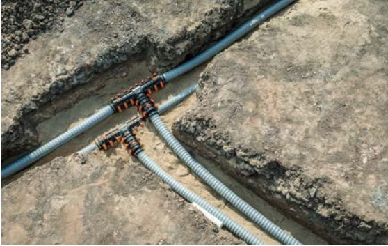
Fig. 07-4 Installation with the trench installation
