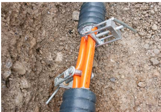
Fig. 07-32 Squeezing off DUO carrier pipes
