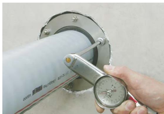
Fig. 05-12 Installation using a torque wrench
