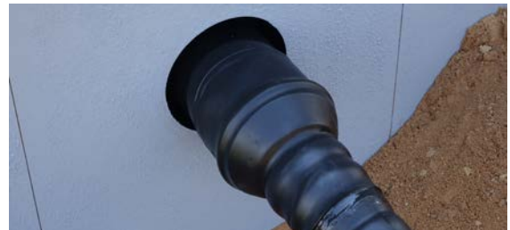
Fig. 05-16 Installation example of a wall entry set with heat-shrink sleeve and link chain seal
