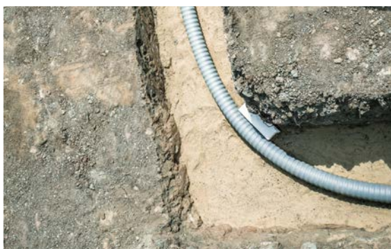
Fig. 07-23 Changes in direction without fittings
