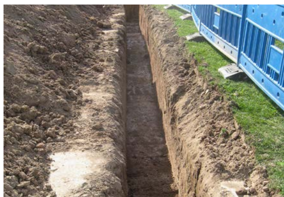
Fig. 07-1 Suitable trench base
