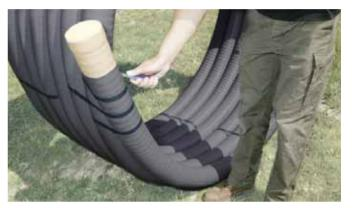
Fig. 44 Cutting the coil straps
