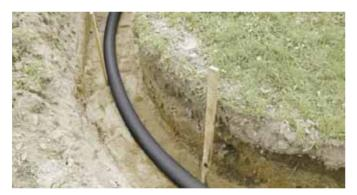
Fig. 47 Laying a bend area
