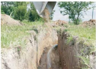
Fig. 49 Backfilling trenches with sand
