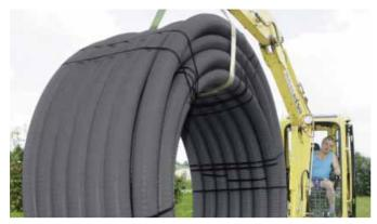
Fig. 40 Lifting with a digger
