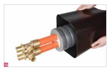
12 Slide the top of the T-Shroud over RAUVITHERM Pipe.
