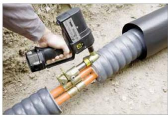
Fig 2 RAUVITHERM compression sleeve joint
