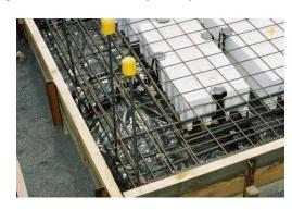
having polystyrene laid in the floor and which give great passive energy storage and are very crack resistant – ideal for polished concrete floors. If your site has more than Im of slope it is not cost effective to use a concrete floor and timber piles can be used, with a wooden floor. If your site is very steep the best design solution is to use poles.
