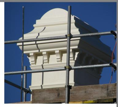
A homestead with a Historic Place Category 2 listing suffered earthquake damage to its ornate Victorian chimney. Due to the home's historical stamp, the chimney required dismantling and rebuilding to its original state.
