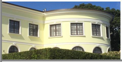
The enormous DecraShape® curved mouldings with dentils measured almost 1.5 metres in height, and were expertly installed by **Andrew** Plastering.
