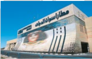
Airport, Assuan, Egypt
