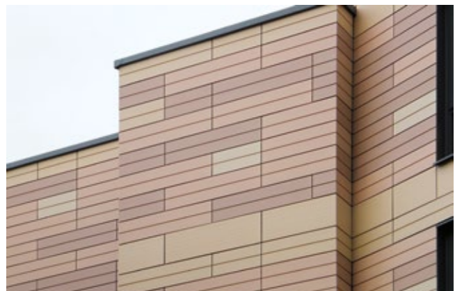
Hall of residence Emmanuel College, Cambridge, Great Britain / Architect: Bidwells / Year: 2016 / Photo: David Salmon
