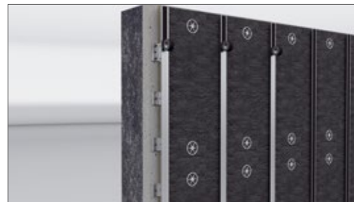
Apply joint tape on vertical bearing profiles
