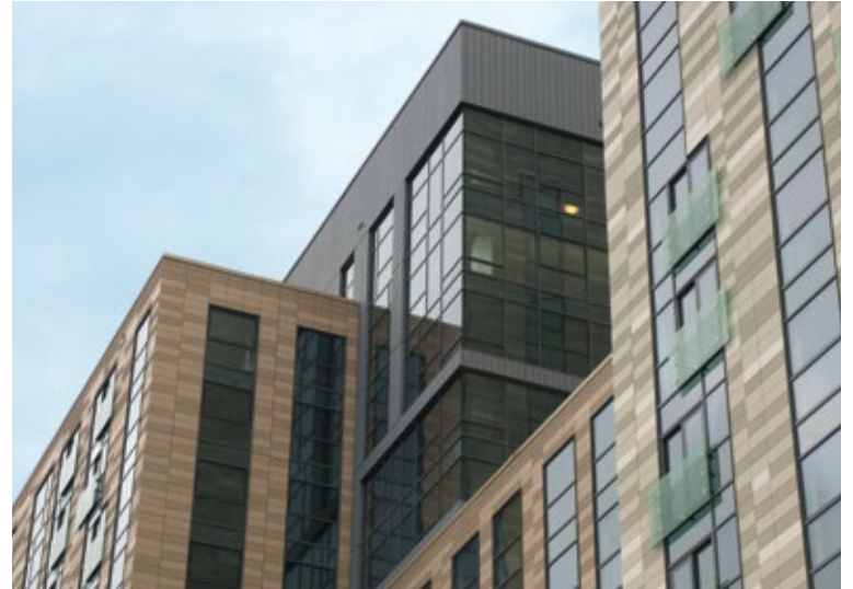
The Viridian, Boston, USA / Architect: Bruner/Cott & Associates Photo: Fred Clements / LEED GOLD
