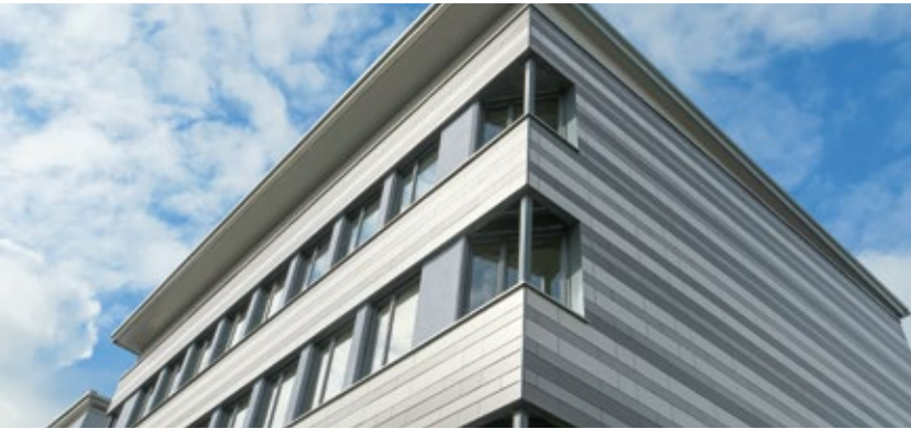
Naabtal-Realschule (secondary school), Nabburg, Germany / Architect: Architekturbüro Schönberger / Year: 2016 / Photo: Atelier Bürger
