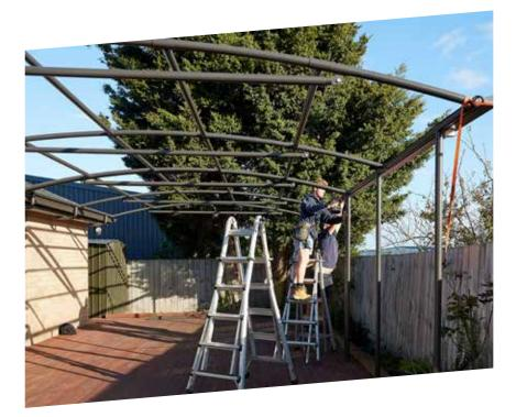
To minimise corrosion and add durability, we apply a two step powder coat system to our pre-galvanised steel. Our powder coating system resists chipping, scratching, and wear, ensuring the frame remains highly resistant to moisture/corrosion creep if damaged. We recommend regular cleaning to maintain the longevity of the frame. Hot dip galvanised finish will be supplied if the property is located in a corrosive environment or near the coast.
