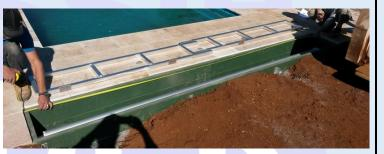
Install gearbox/motor - Install roller end mount and roller tube - Measure and trim as appropriate
