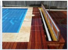
Install the lid frame - apply lid frame cover material (ie decking boards) - install the pool cover
