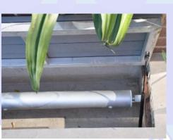
measure, trim (if required) and install lid frame - Install gearbox, end mount and tube assembly
