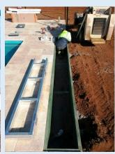
Excavate & build frame using framing brackets - Install frame to desired level, concrete in place, set paving
