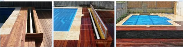
Install the lid frame - apply lid frame cover material (ie decking boards) - install the pool cover
