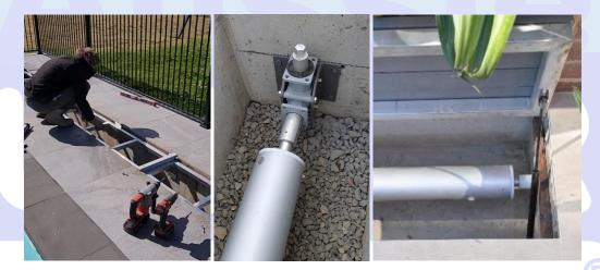
measure, trim (if required) and install lid frame - Install gearbox, end mount and tube assembly
