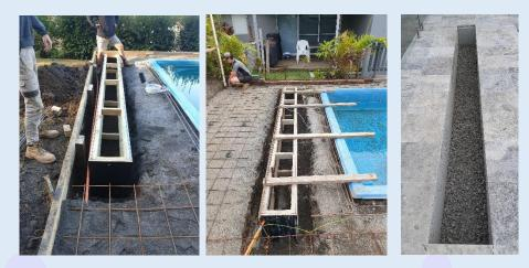
Form pit - allow suitable drainage – install finished surface (concrete, tiles or pavers)
