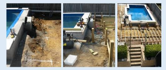
Layout deck to accommodate the opening required for the kit – refer to plan provided with kit Formal drain or gravel pit and agi line may be appropriate drainage
