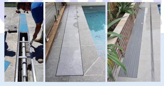
Install chosen lid frame covering ie. decking, composite decking or tiles - install pool cover
