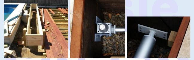
Install framing to create the deck opening required for the kit - mount gearbox, end mount and tube assembly
