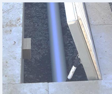
7.5mm Blueboard/Villaboard and 12mm tile on lid frame
