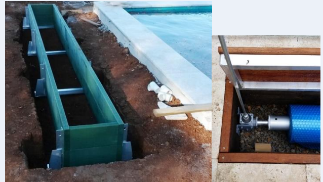
In-ground installation using framing brackets
