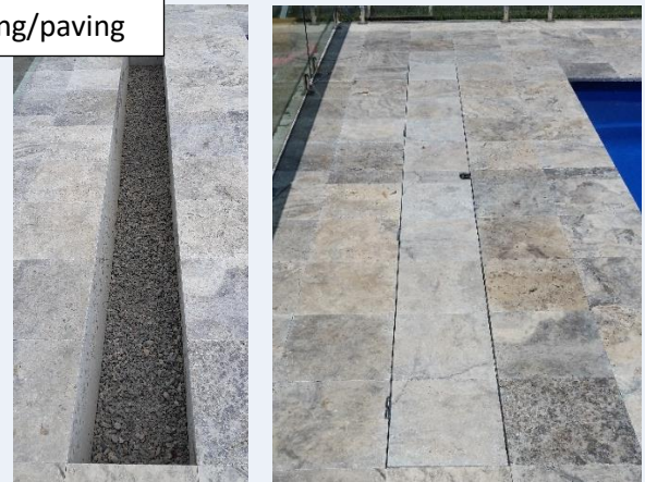
Concrete Pit installation
