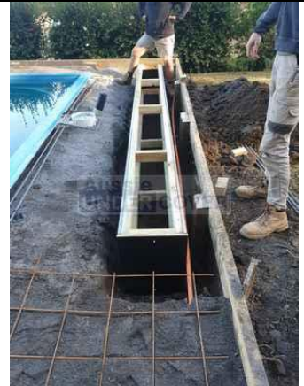
N12 rio in all walls & corners top and bottom
