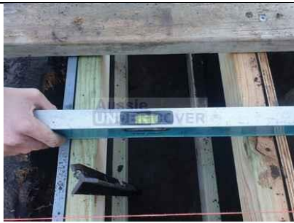
Timber brace attached to formwork and pool edge to stop movement during concrete pour
