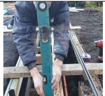
Timber brace attached to formwork and pool edge to stop movement during concrete pour
