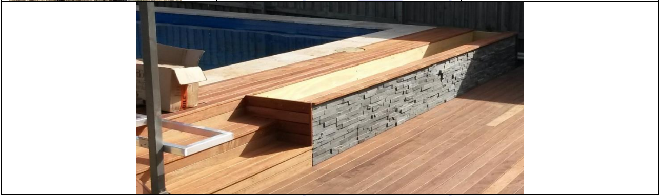
Cavity lining 190 x 35 or 245 x 35 as required
