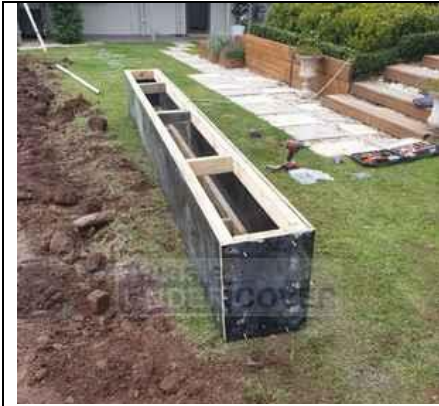
Overall completed formwork = Pit length by 390mm wide x 450/500mm high/deep
