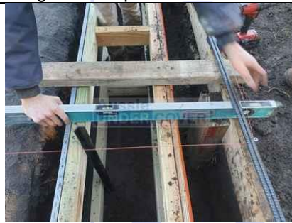
Timber brace attached to formwork and pool edge to stop movement during concrete pour
