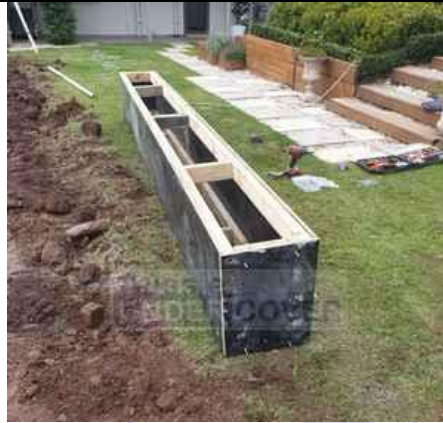
Completed form work 390mm wide x 500mm deep Length to suit pool & kit
