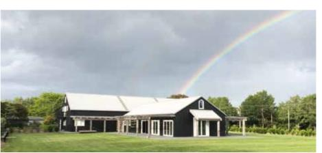
Building regulations meant he couldn't stain the timber; it had to be painted. He chose Resene's 'All Black' for the timber cladding, which contrasts with the lighter Colorsteel Endura 'Sandstone Grey' roofing. The paint is one of Resene's CoolColour range, specially formulated for dark paints so that they don't absorb as much heat, which can cause the paint to fail and lead to cracking and cupping of timber.
