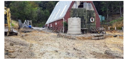
Boat Yard Remediation Validation, Opua
