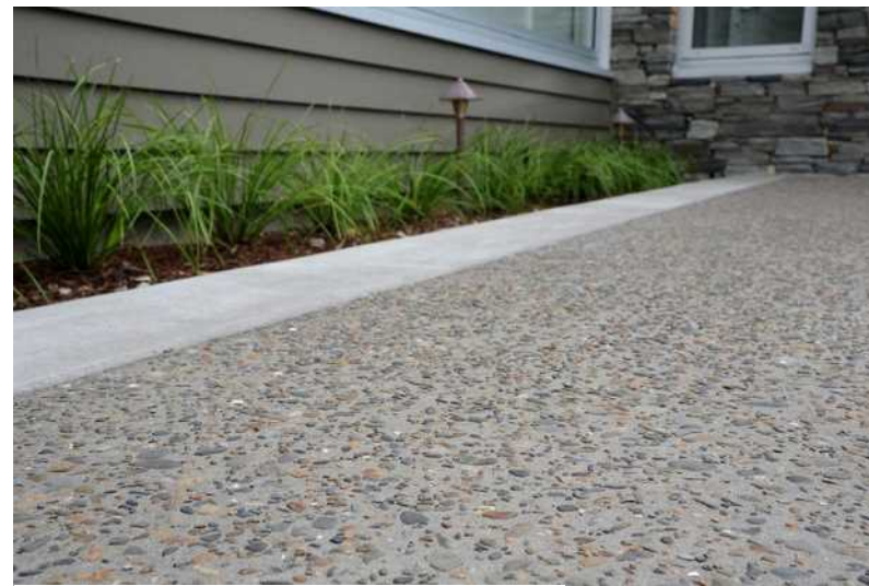
DECORATIVE CONCRETE DRIVE
