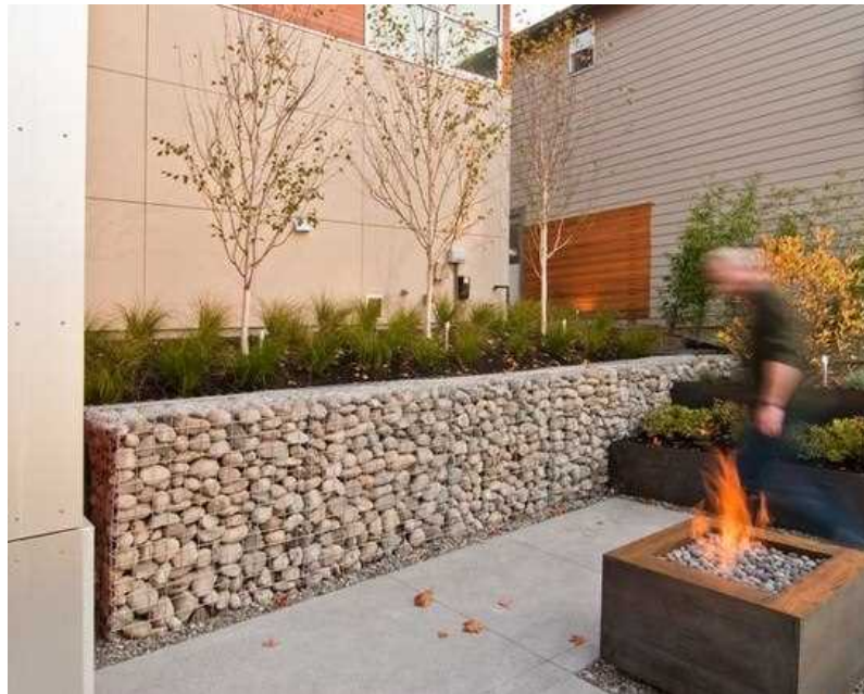
RIVERSTONE GABION BASKET RETAINING
