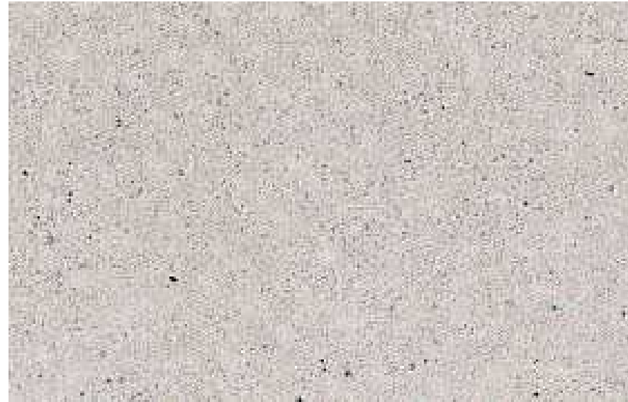
ACID ETCH CONCRETE DRIVE SURFACE
