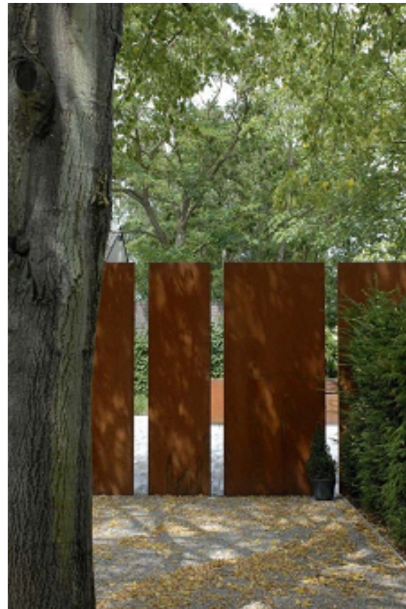
CORTEN STEEL PANELS FOR SCREENING INTERNAL AREAS
