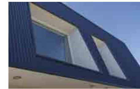
Left: Windows are recessed to reduce the impact of summer sun; Below: A retractable awning allows winter sun in and reduces its intensity in summer; Bottom left: Energy-efficient appliances and lots of natural light reduce power consumption
