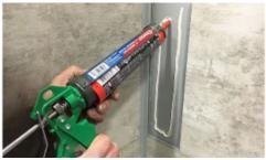
After cutting tile to length, apply adhesive to the substrate, as shown. Spray a squirt or two of water onto the substrate and adhesive, as shown. This will lubricate the substrate allowing for easier movement.
