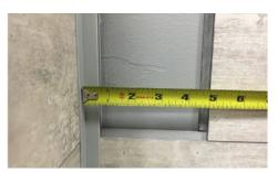
Next, determine the length of the tile section. Measure from the inside lip of the previously installed tile to the inside edge of the pre-installed trim. See image at left for details. In this case, the length to cut the final tile in the row is 101.6 mm (as shown).
