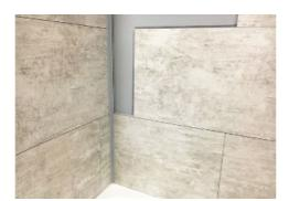
Short tile piece needed to finish row on an inside corner
