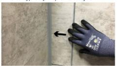
5. Apply sealant to the interlocking edges if this installation is for a wet environment. For further details refer to the Dumawall Installation and follow the sealer manufacturers guidelines. The tile can now be manually pulled into place. Pull the tile toward the interlocking joint. If necessary, rubber gloves can be used to increase grip friction with the surface of the tile. See image below. Keep pulling until the interlocking joint is tight. Pull tile into interlocking joints.
