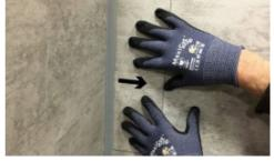
Interlocking joints at tile's right and bottom are tight. Use a damp rag or paper towel to clean off any sealant or adhesive that may have been squeezed onto the tile surface.
