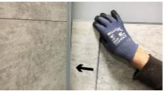
Insert cut end into edge trim channel while holding other edge up. Push the tile into the edge trim while laying the tile down toward the substrate. When pushed into the trim entirely, the interlocking edges will be exposed.
