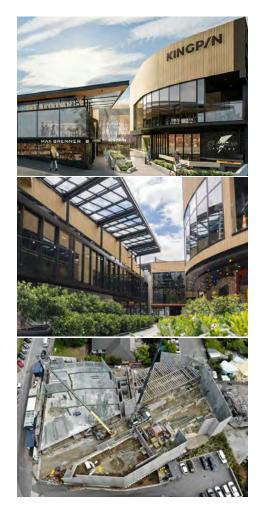
A very restricted brown field site with three dimensional co-ordination of the external services requiring construction sequencing and earthworks to be resolved during design.
