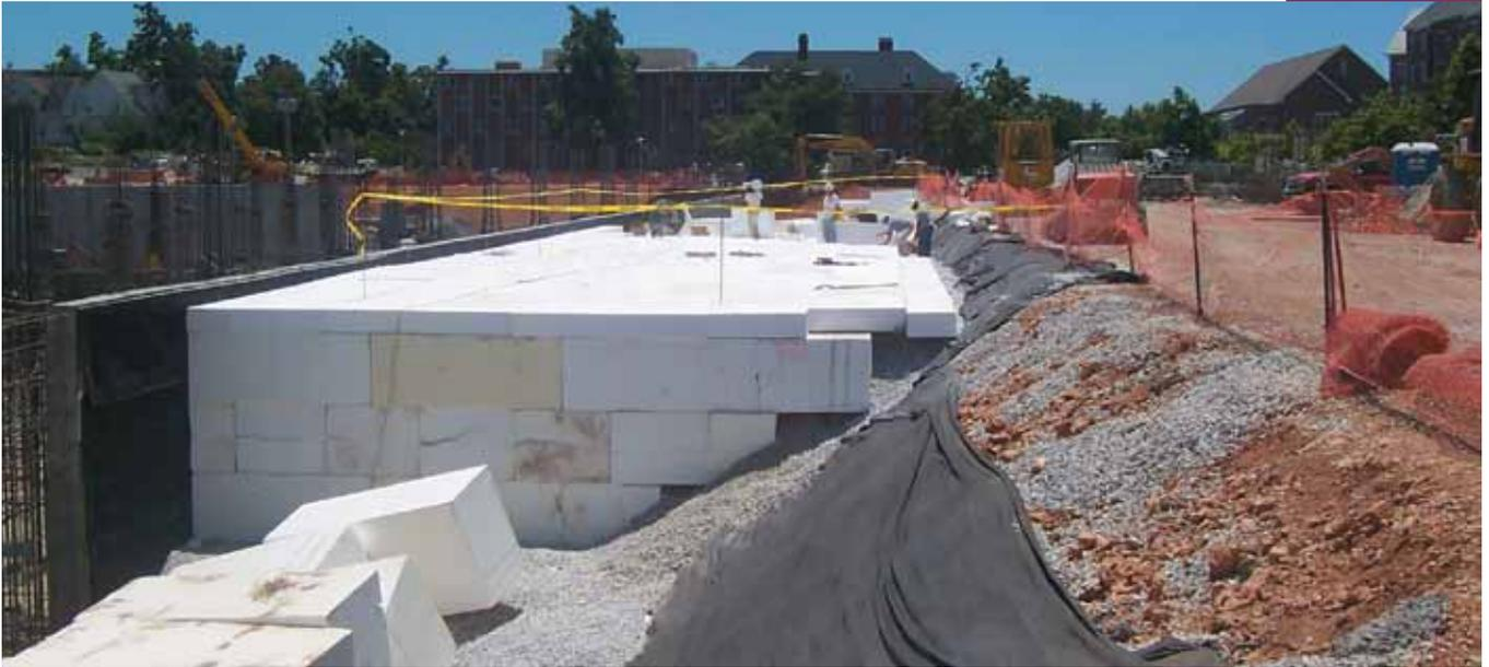
EXPOL GeoFoam can be used as backfill behind retaining and buried structures to greatly reduce lateral pressures on the structure. Because the horizontal pressure acting on a retaining wall is proportional to the weight of the backfill, a less robust retaining structure is needed if the backfill soil in the active zone behind the retaining wall is replaced with EXPOL GeoFoam.
