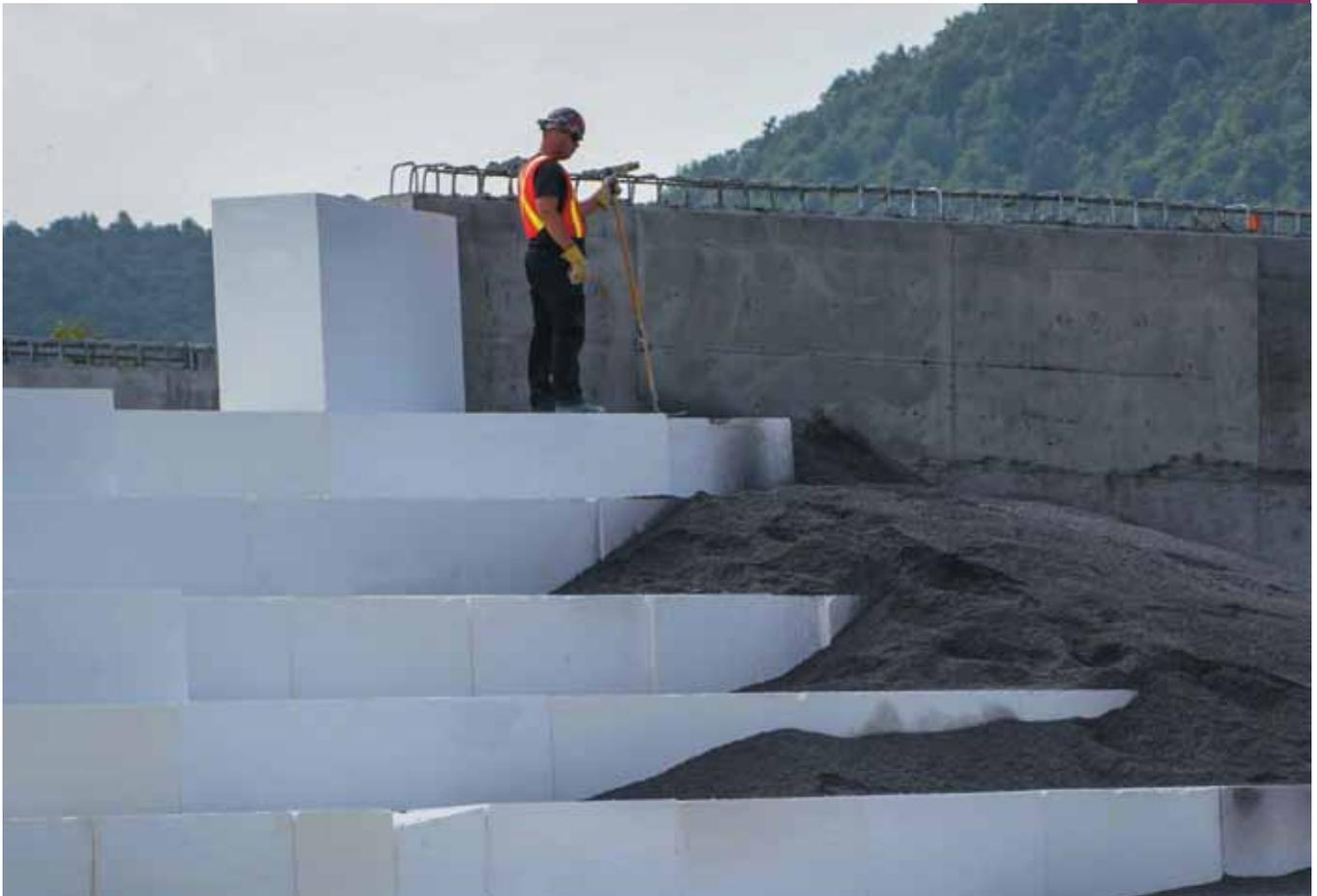
There are several advantages to using EXPOL GeoFoam to construct approach fills for bridge abutments. Because of its high compressive resistance, EXPOL GeoFoam can safely support highway loading without over-stressing the underlying soils. This usually results in less differential movement at the bridge/approach fill interface, which reduces the construction cost of the approach slab and its long-term maintenance. In addition, when compared to traditional embankment
