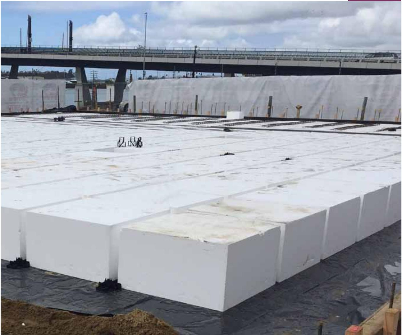
EXPOL GeoFoam is often used in raft type pod floors. The combination of deep and thicker concrete ribs along with high density polystyrene pods creates a highly engineered foundation (See table page 13). The pods are cut to size to suit each particular project however to
