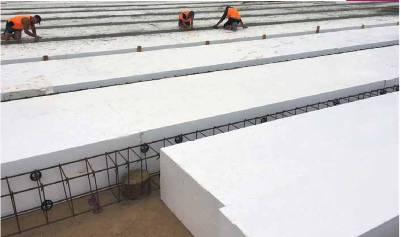
EXPOL GeoFoam can be used as a compensating foundation to reduce the load on underlying compressible soils and minimize building settlement along with potential bearing capacity problems. Existing soil is excavated to reduce the net applied load to the soil
