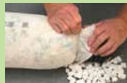
Push sleeve and polystyrene down pipe to required length. Re-tie with new cable tie supplied, trim excess sleeve off
