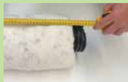
Measure the length required
