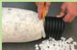
Cut the cable tie and remove excess polystyrene
