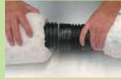
Push sleeve and polystyrene down pipe to required length. Re-tie with new cable tie supplied, trim excess sleeve off
