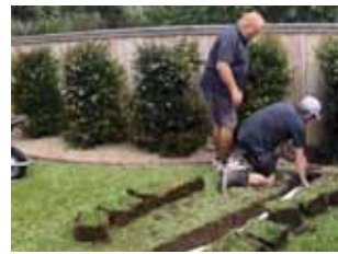
3. Lay QuickDrain
