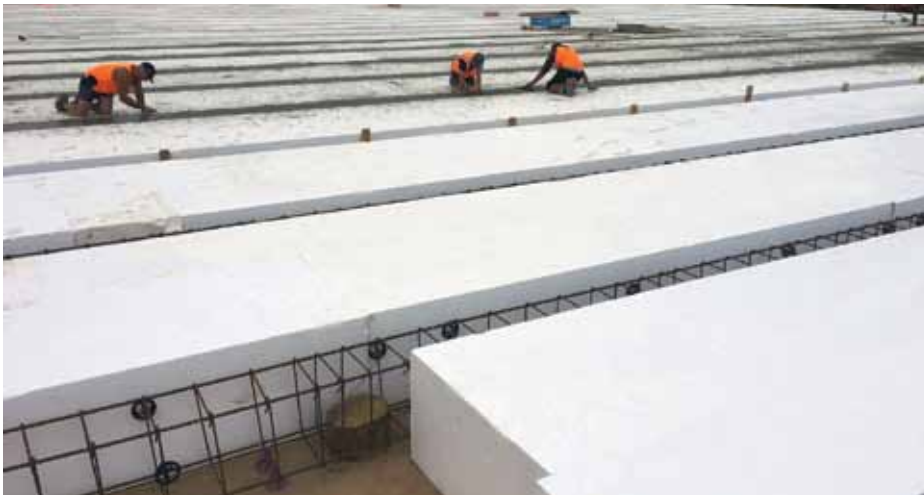
EXPOL GeoFoam as lightweight fill under a concrete floor
