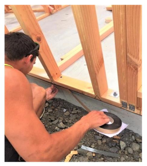
Only apply FPS Butyl DS Tape to clean, dry and stable concrete or timber foundations. If the concrete foundation is very rough or has severe indentations – apply 2 or more layers of FPS Butyl DS Tape to these imperfections. For brick veneer cladding, apply FPS Butyl DS Tape after rebate sealant has been applied and dried.
