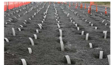
PJK Expressway, Wick Drains
