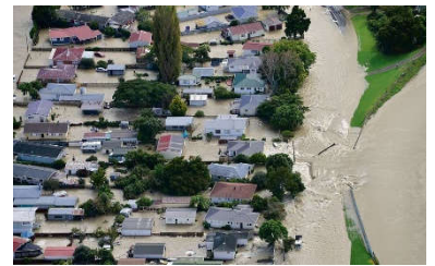
Edgumbe, Stopbank Failure
