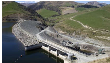
Opuha Dam, South Canterbury
