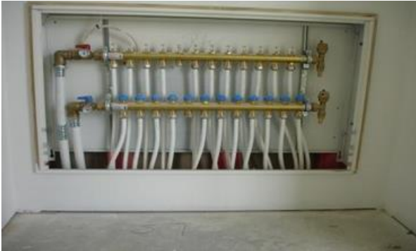
Underfloor Heating Manifold
