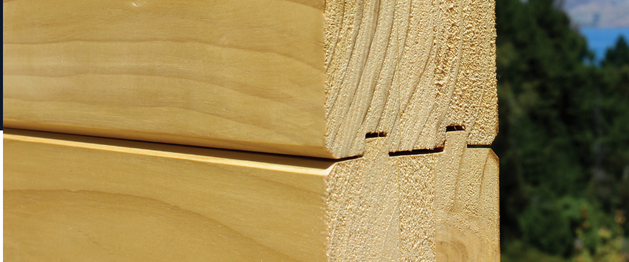
Interlocking walls (internal walls shown) in a Fraemohs Solid Timber home. Our timber provides the internal finish, external finish, insulation, and structural strength. Just wood. No trickery.
