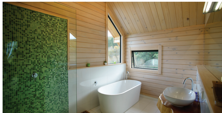
If you look carefully in this picture you can see that the shower, bath mixer and vanity are framed off the Solid Timber wall. This allows space for the plumbing to come up through the floor behind these fixtures
