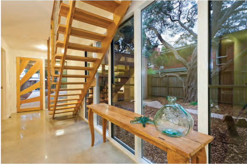
➦ The staircase was crafted by Coastal Staircases Geelong from recycled messmate flooring joists. Beside it, full length low-e double-glazed windows provide a visual connection to the treed site.
