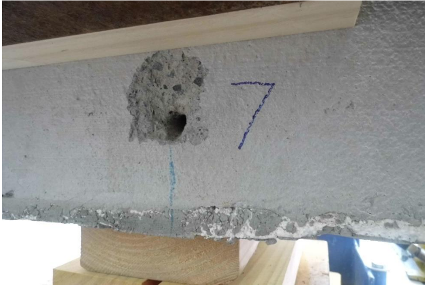
Photograph 10. Concrete cone failure under tension loading
