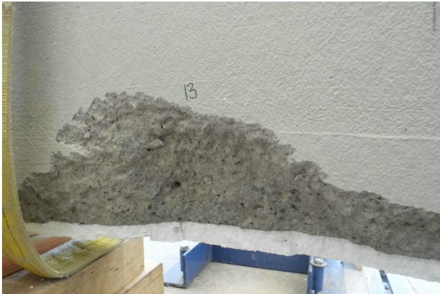
Photograph 11. Concrete edge breakout under tension loading.
