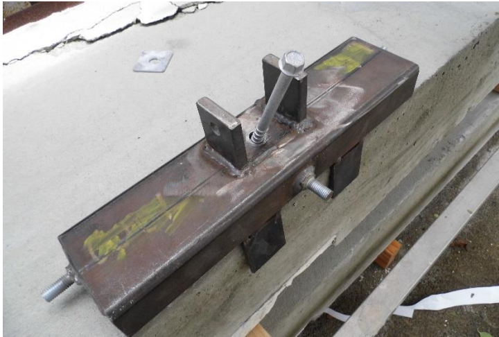
Photograph 3. Jig used for drilling pilot hole for anchor.
