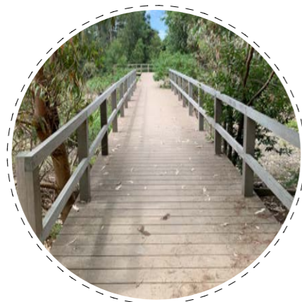
EXISTING TIMBER PLATFORM
