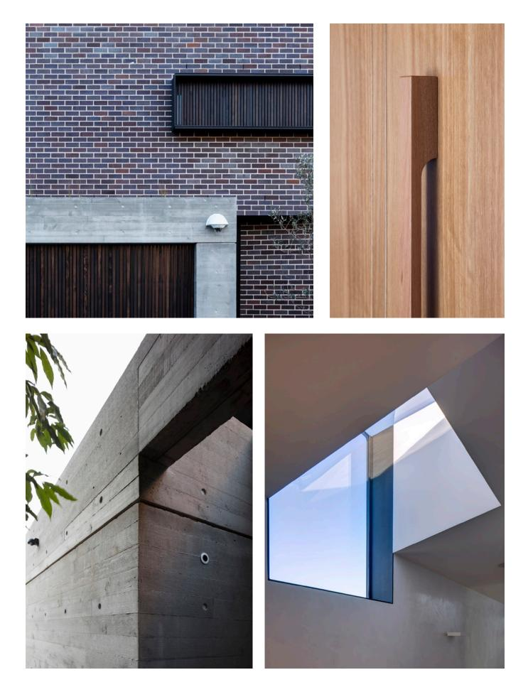
From a building perspective this project was complex, and required a high degree of foresight and team collaboration, as elements such as formwork, brickwork and bespoke windows were designed to be exposed – thus requiring incredible attention to detail at every stage. The quality of craftsmanship and construction are on show for all to see and this was one of the major challenges of the build – It had to be built right the first time.
