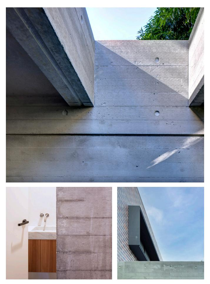
The concrete formwork was designed to be an architectural element, which meant that we had to pay complete attention to to the final form in every process. Consideration to material junctions such as the expressed steel and brickwork was essential to align the textured imprints of the the concrete around the building. The end result was beautiful architecturally, making it obvious that consideration and care had been applied throughout.
