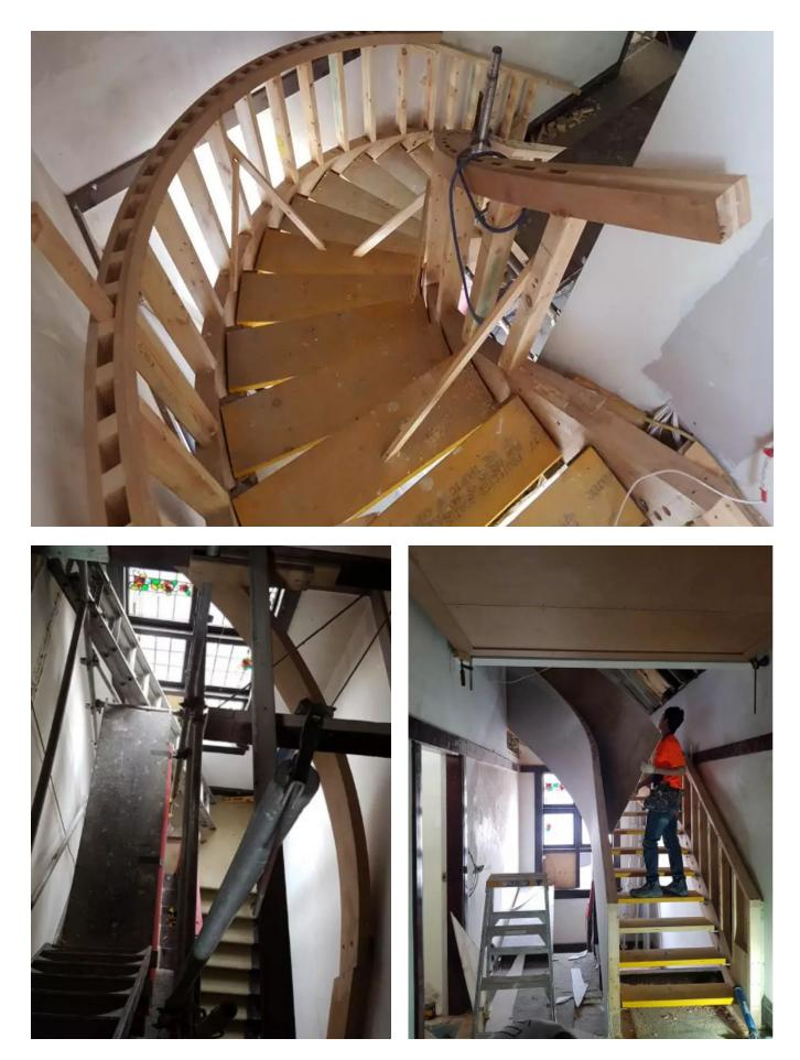
The staircase presented its own challenges. We needed to execute a tight sweeping radius that provided clearance to the raked roof above and existing stairs below. Our initial intention was to use steel, however stability could not be achieved.
