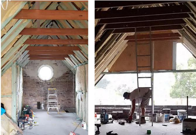
From a building perspective this posed the challenge of maintaining the design integrity, whilst providing complete stability within the existing roof structure. The existing roof framing was reinforced with a new frame structure to withstand the removal of supporting members. A further sub-frame structure was then required to achieve the design intent for the placement of overhead beams and raked linings.
