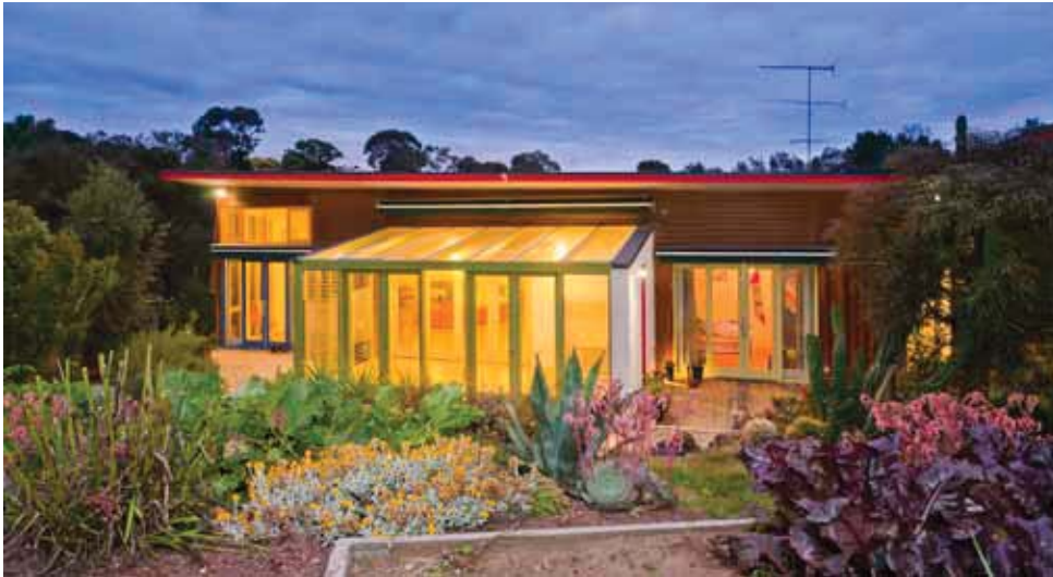
These images show the automated motorised awnings on the northern facade, and how they work to shade the wintergarten and slab in the heat of summer.
