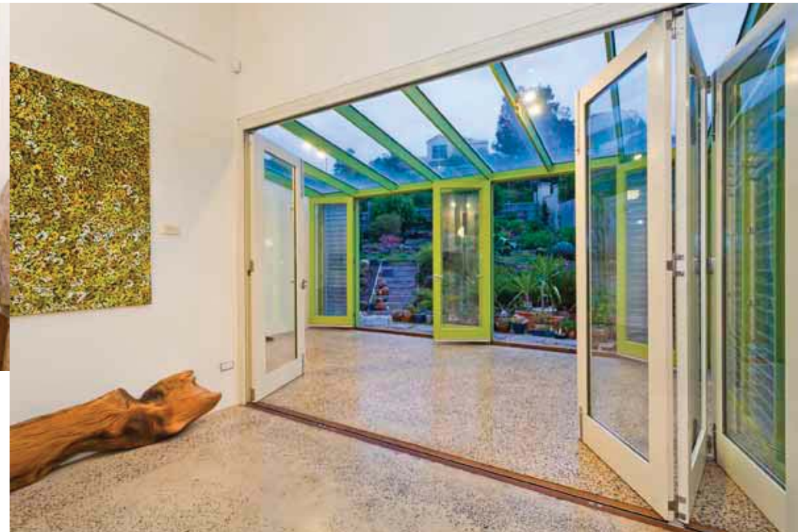
These images show the wintergarten at work. From left to right: Jan and Anne keep the wintergarten fully closed on a hot summer's day or winter night to keep heat out (summer) or in (winter); during winter they open the internal double-glazed doors, letting the air that has been captured and heated by the slab in the wintergarten into the living and dining room; on a summer's night both the internal and external doors can be opened to encourage cooling cross ventilation through the house and to allow the concrete slab in the wintergarten to cool.
