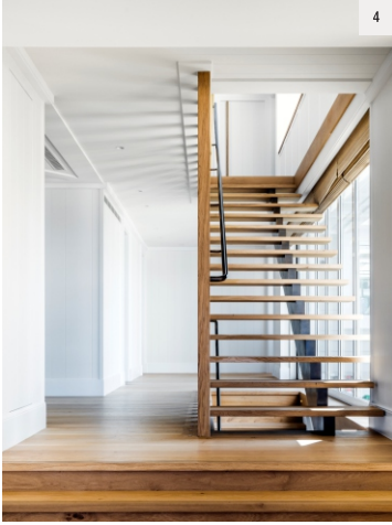
▼ IMAGE NO 4 Open Riser Staircase
