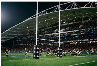
North Harbour Stadium, Albany
