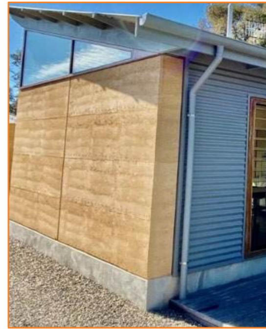
Figure 1 - Example of an RE wall with exposed edgebeam and window over showing shrinkage joint. Photo courtesy of https://www.aseg.net/rammed-earth-building-gallery/
