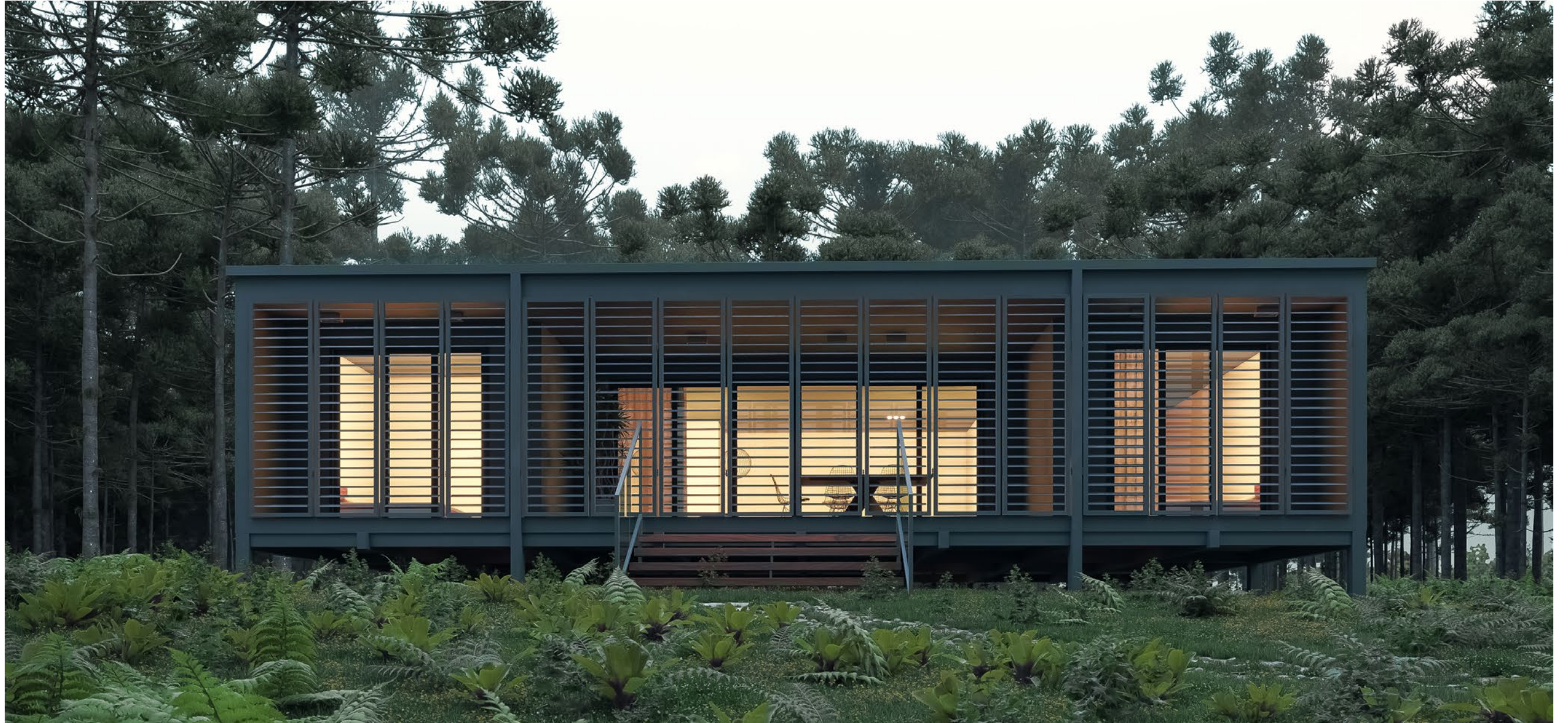
Project Name: Mangawhai Lodge | Client: Future House NZ Limited | Location: Mangawhai, New Zealand
