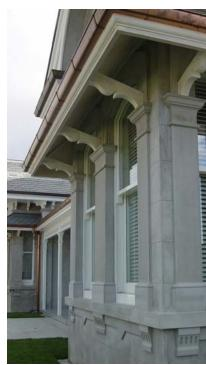
Using our strong lightweight material with KickIt® plaster, we were able to create the capitals, bangles, tapered half columns, plinths, sills and decorative details underneath the sills.
