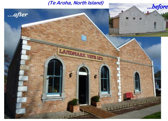
This historical building with majestic mouldings was originally constructed in 1884. Due to 128 years of exposure to the elements, the building was completely dismantled and reconstructed, including using some of the original bricks.
